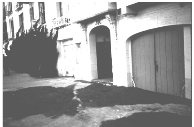
Figure 40 - Loma Prieta Earthquake, October 17, 1989. Lateral spreading, liquefaction and sand boils caused extensive damage in the Marina District of San Francisco, about 60 miles away from the epicenter.
